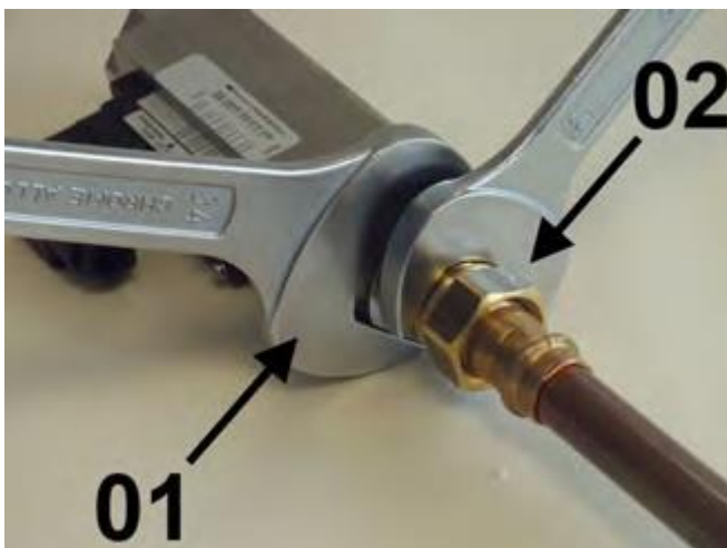
Fig. 11 Screw in the device
